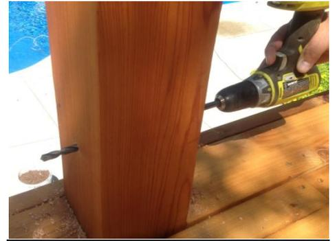
Drilling hole through post to prep for bottom brackets install
