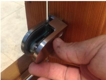
Pushing the 2nd half of bracket onto installed half of bracket.
