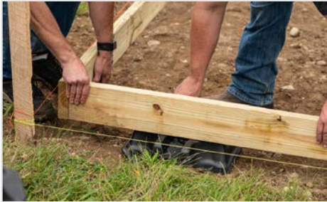
PLACE BLOCK PIERS AT THE CORNERS OF YOUR PROJECT.
