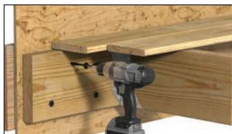
LEDGER BOARD CONNECTIONS
